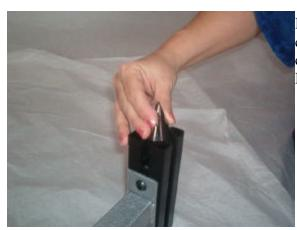
Install a setscrew into each of the cones. Install a cone onto each of the columns. Note: Don't leave cones sitting around with the point facing upward. If a person fell onto one it would hurt.
